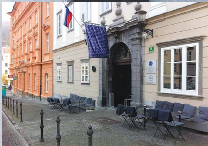
Central building of the Scientific Research Centre in the Slovenian Academy of Sciences and Arts building at Novi trg 2
